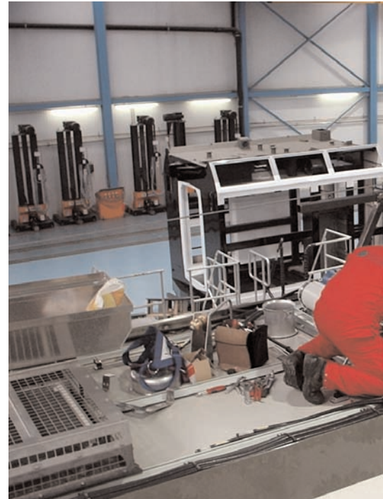
Installation during ongoing production
